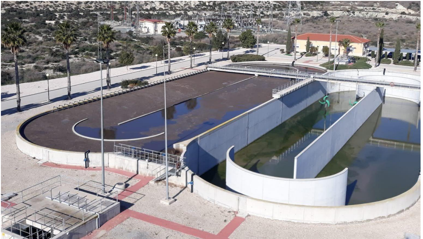
WWTP of Cieza (Murcia) – Biological reactor
