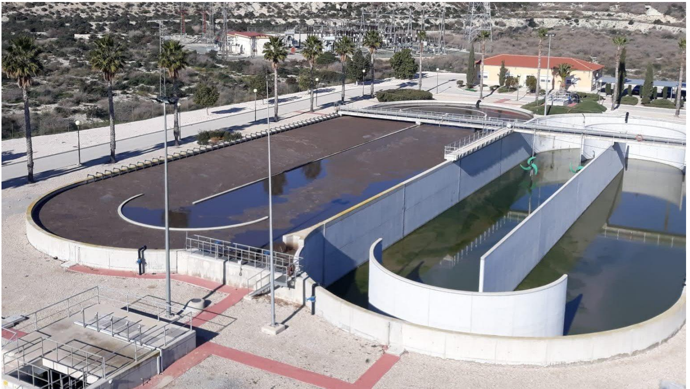
WWTP of Cieza (Murcia) – Biological reactor
